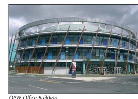
OPW Office Building
