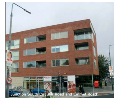
Junction South Circular Road and Emmet Road
