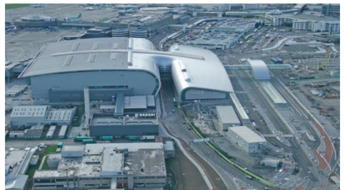
New Terminal 2 at Dublin Airport
